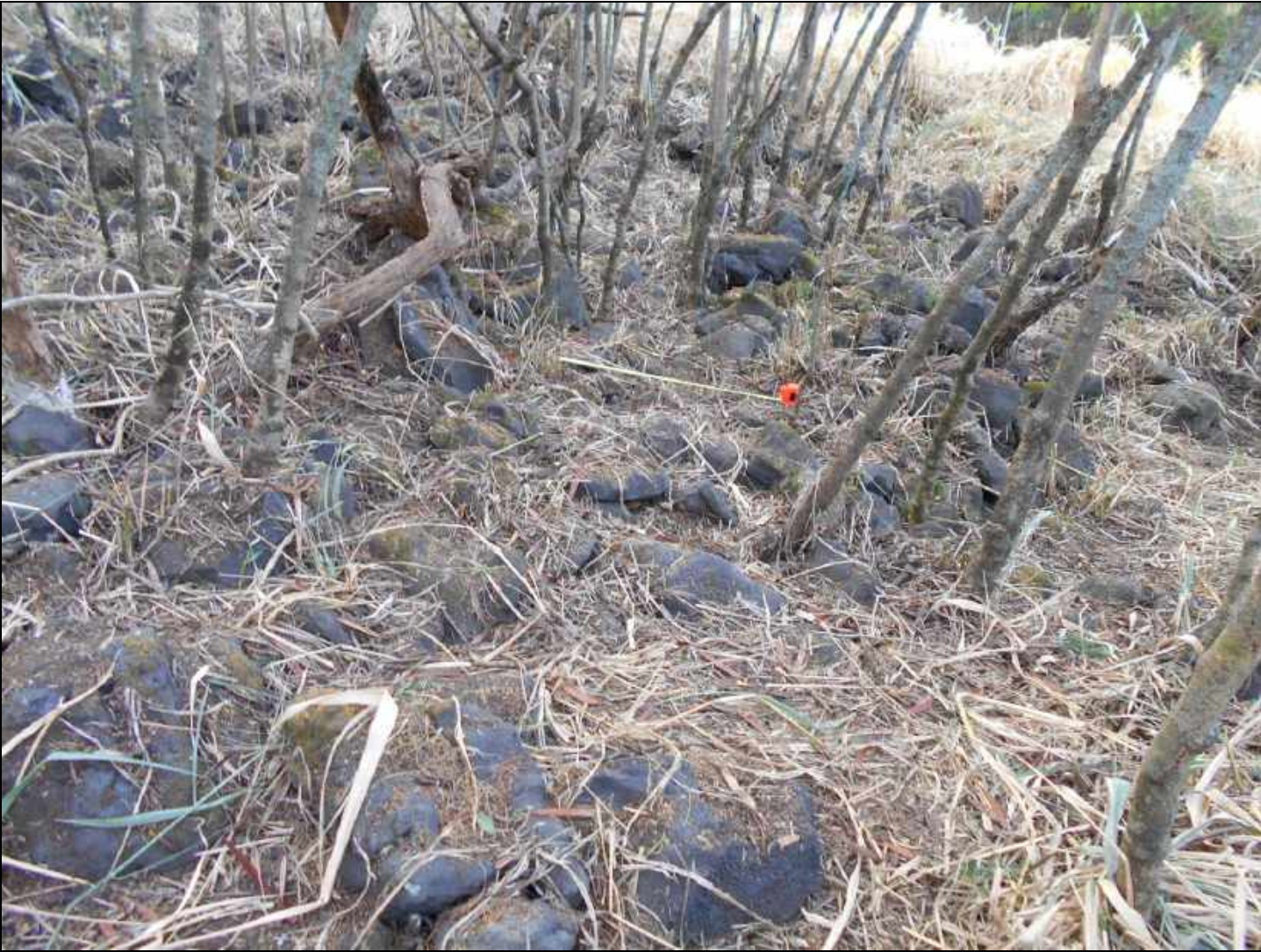
Figure 70: Photograph of Site 30607 Feature 5 Looking South.
