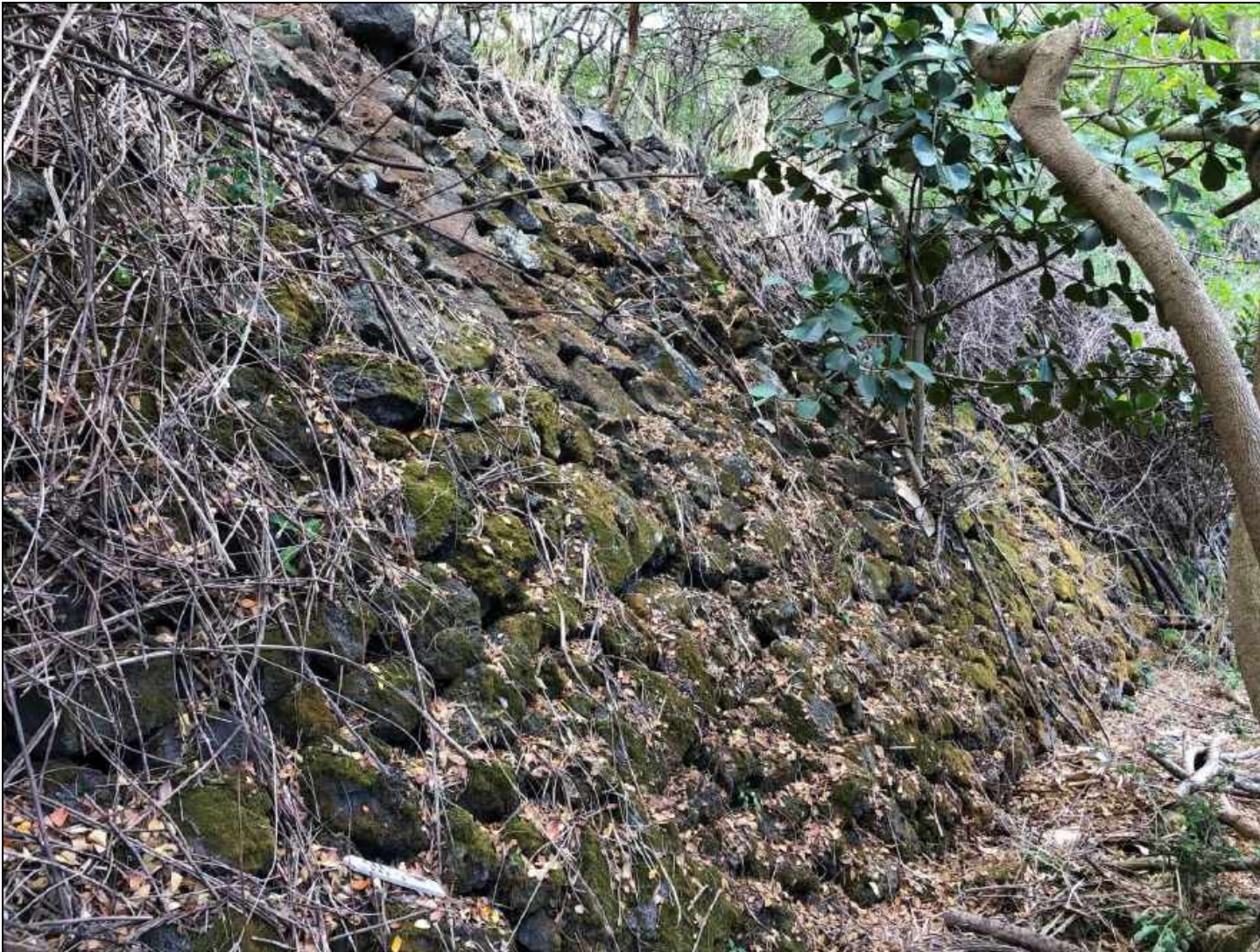
Figure 13: Photograph of Site 30592 Railroad Berm Retaining Wall, Looking Southeast.
