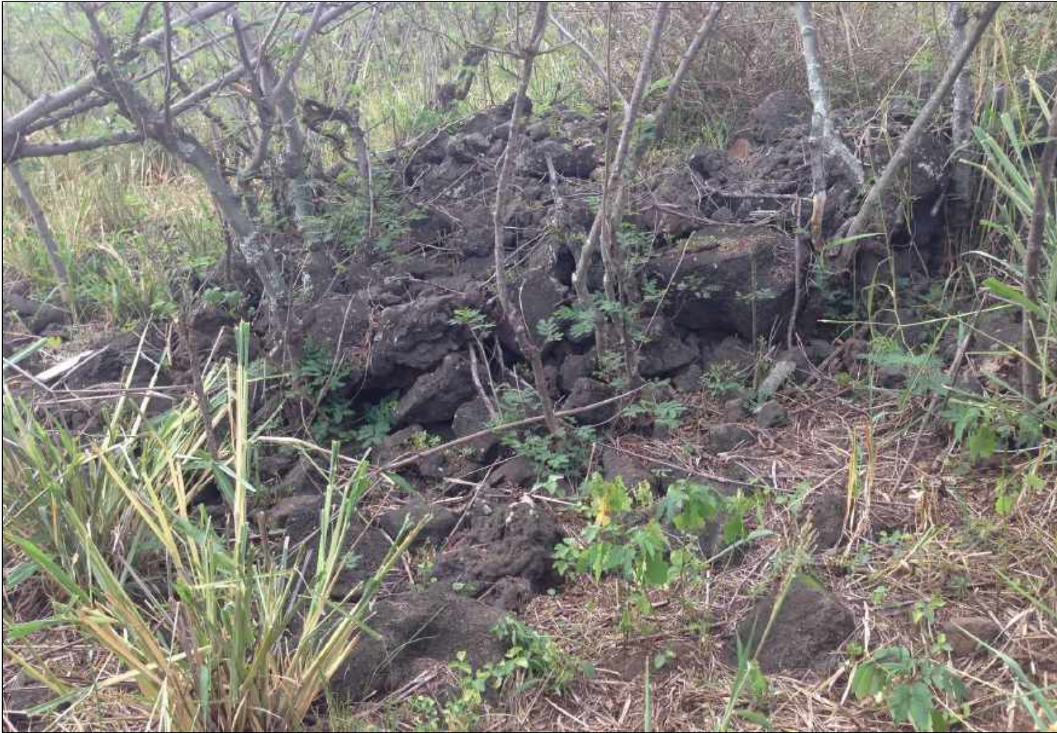
Figure 24: Photograph of Site 10013 Enclosure South Corner and West Wall, Looking Northwest.
