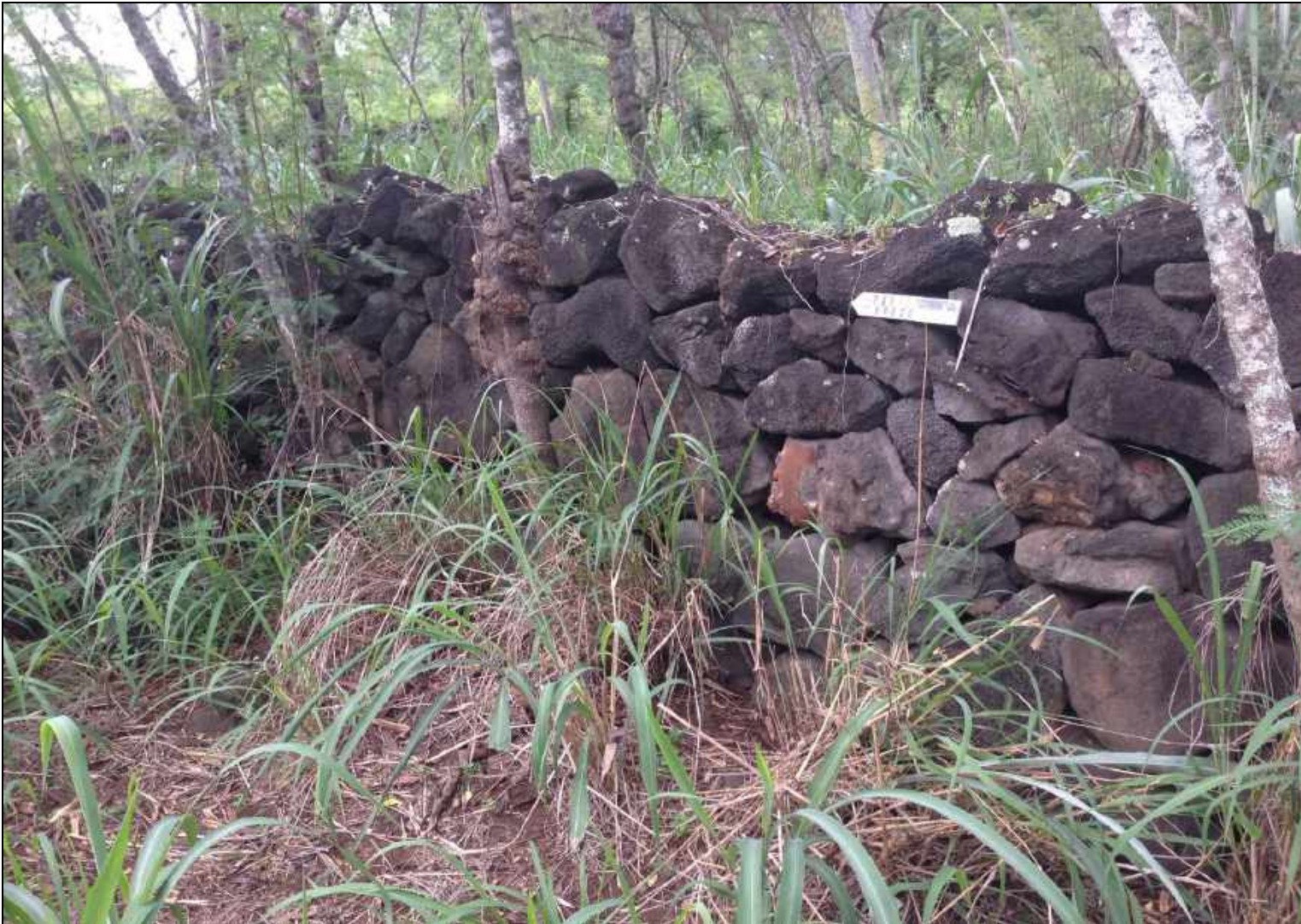
Figure 71: Photograph of Site 31182 Feature 11 Showing Wall Construction, Looking East.
