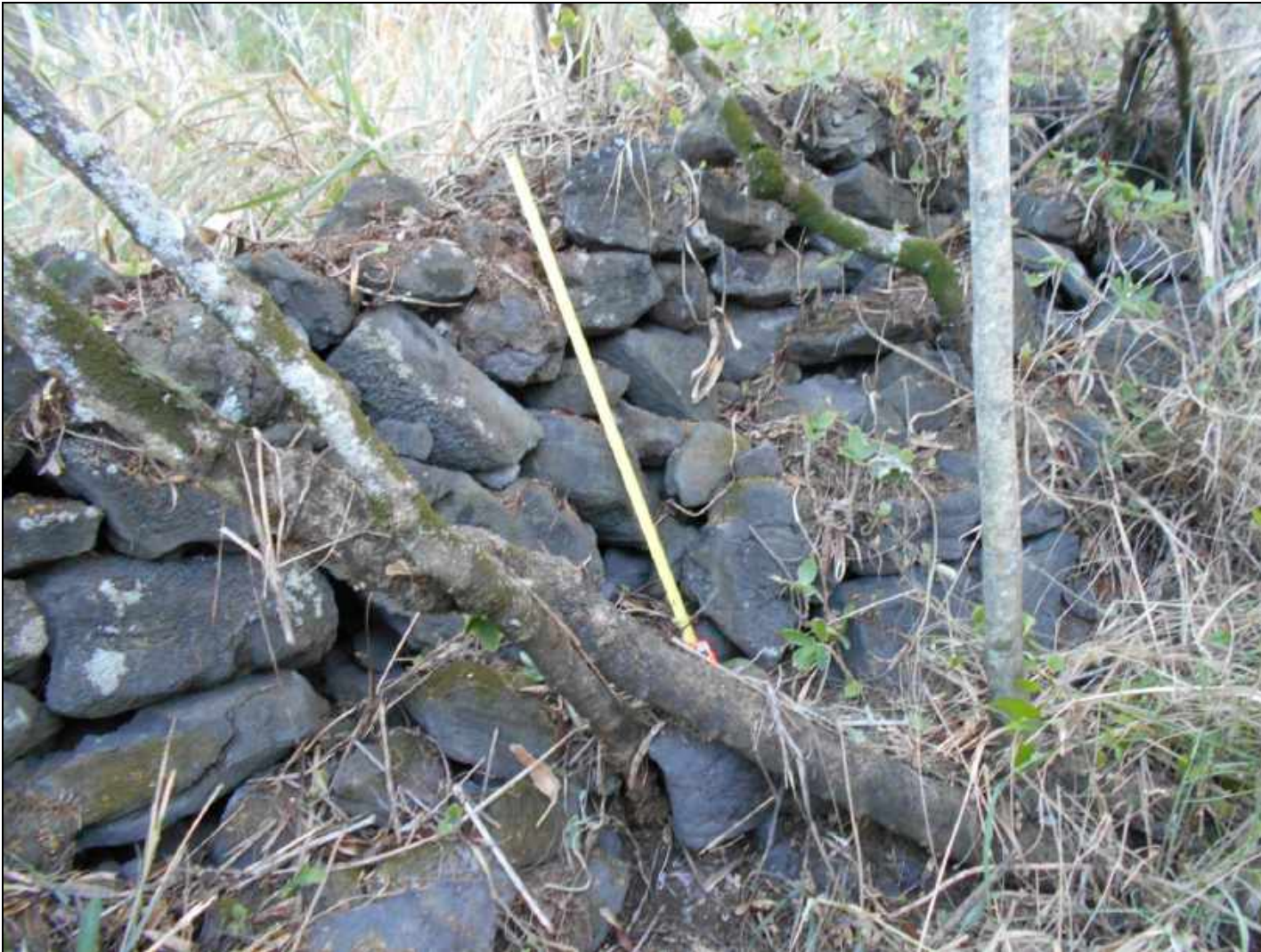
Figure 60: Photograph of Site 30605 Wall Looking Northeast.
