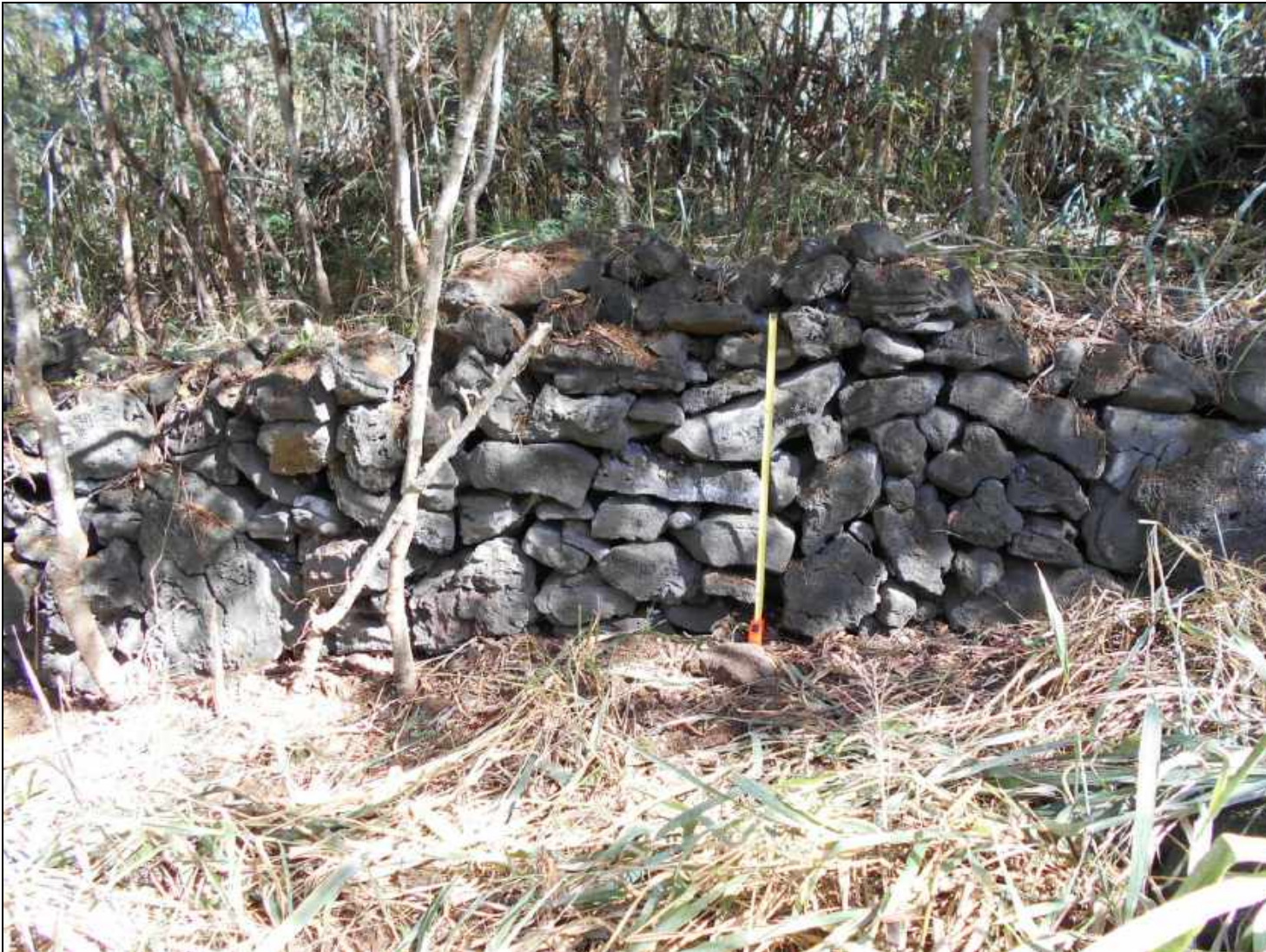
Figure 26: Photograph of Site 30595 Wall Looking North.
