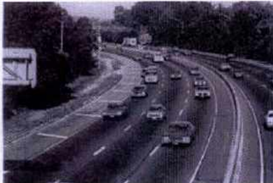
Level of Service B: Stable traffic flow with a high degree of freedom to select speed and operating conditions but with some influence from other users.
