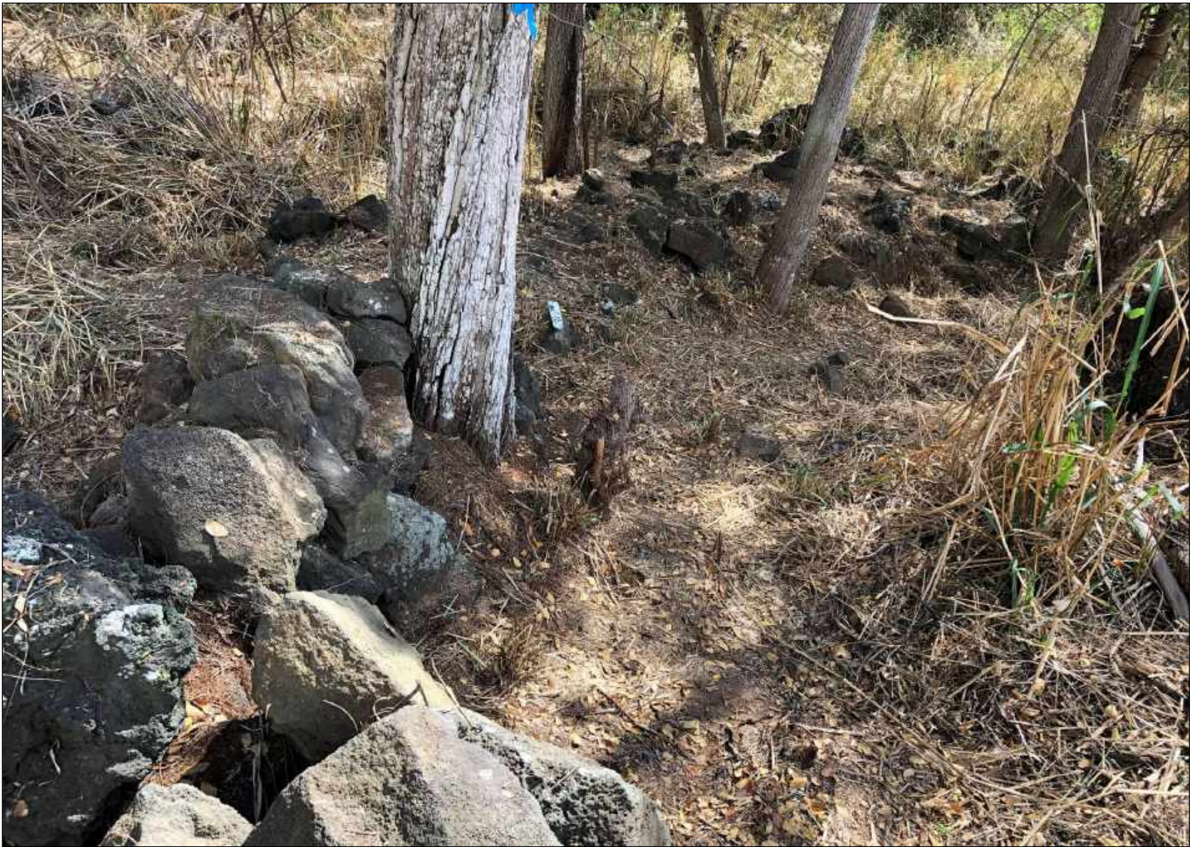
Figure 54: Photograph of Site 10074 Rock Wall, Looking South.
