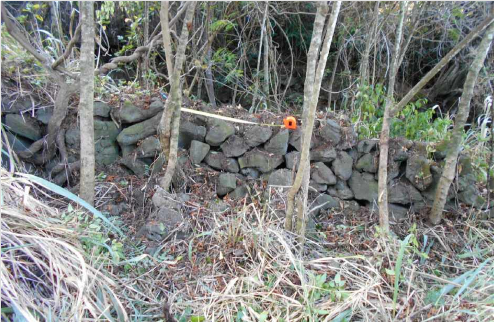
Figure 33: Photograph of Site 30597 Wall with Gulch in Background, Looking South.
