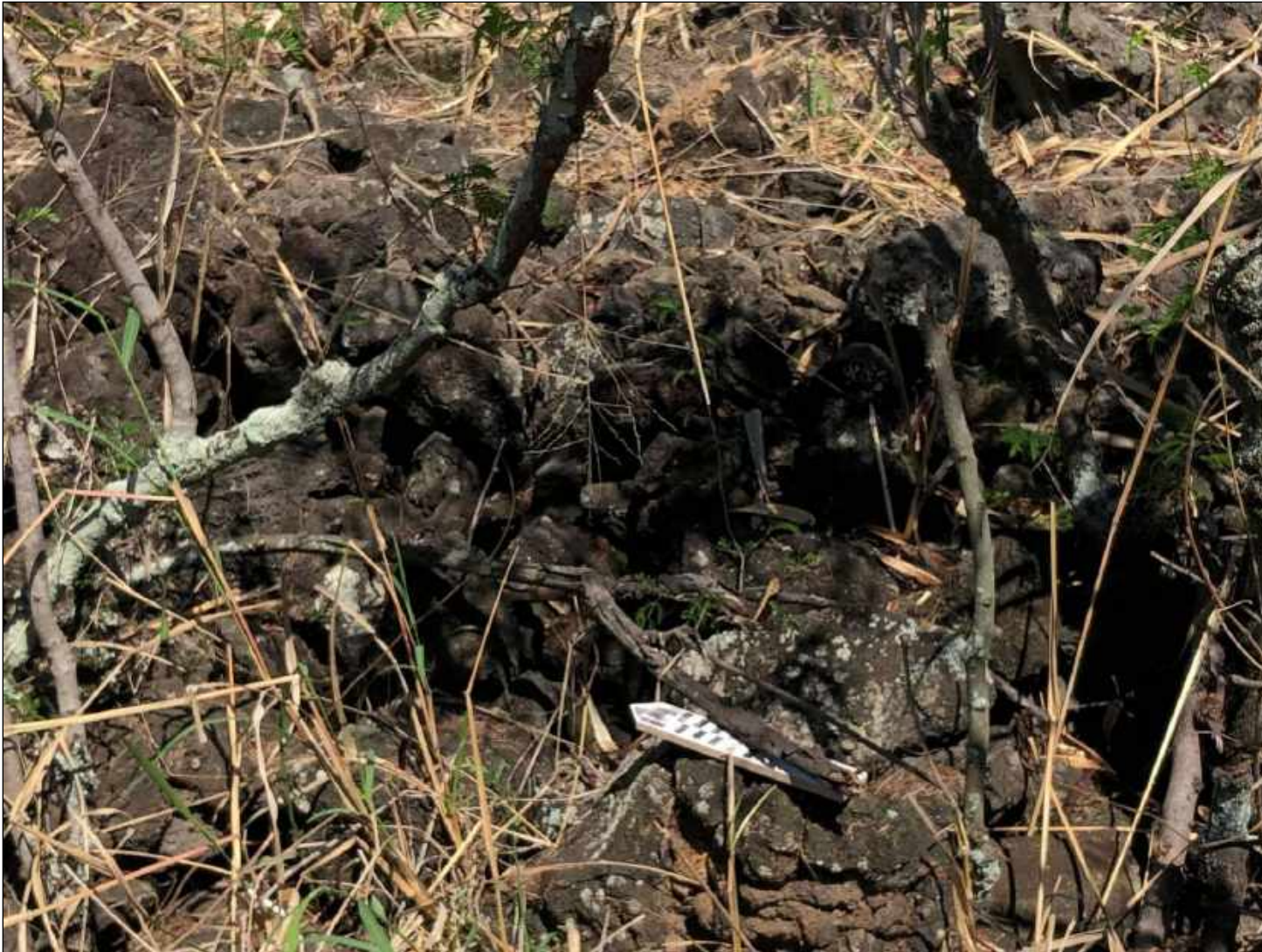
Figure 17: Photograph of Site 10011 West Edge Construction and Collapse, Looking Northeast.
