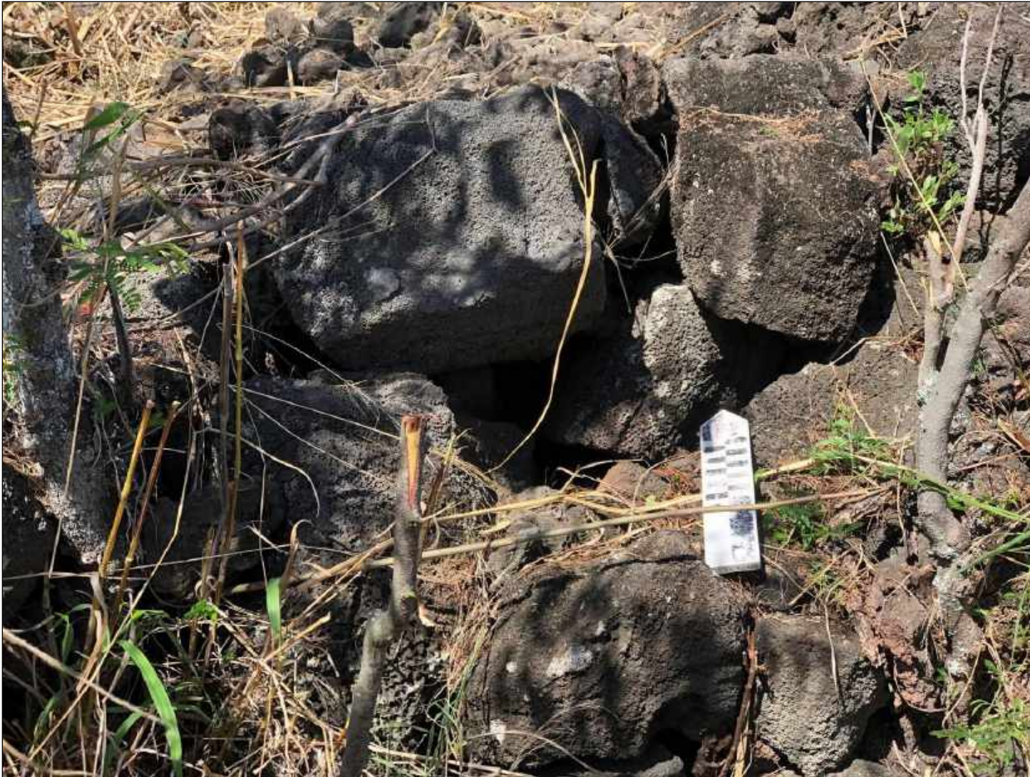
Figure 16: Photograph of Site 10011 South Edge Construction, Looking North.
