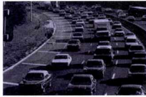
Level of Service F: Forced traffic flow in which the amount of traffic approaching a point exceeds the amount that can be served. LOS F is characterized by stop-and-go waves, poor travel times, low comfort and convenience, and increased accident exposure.
