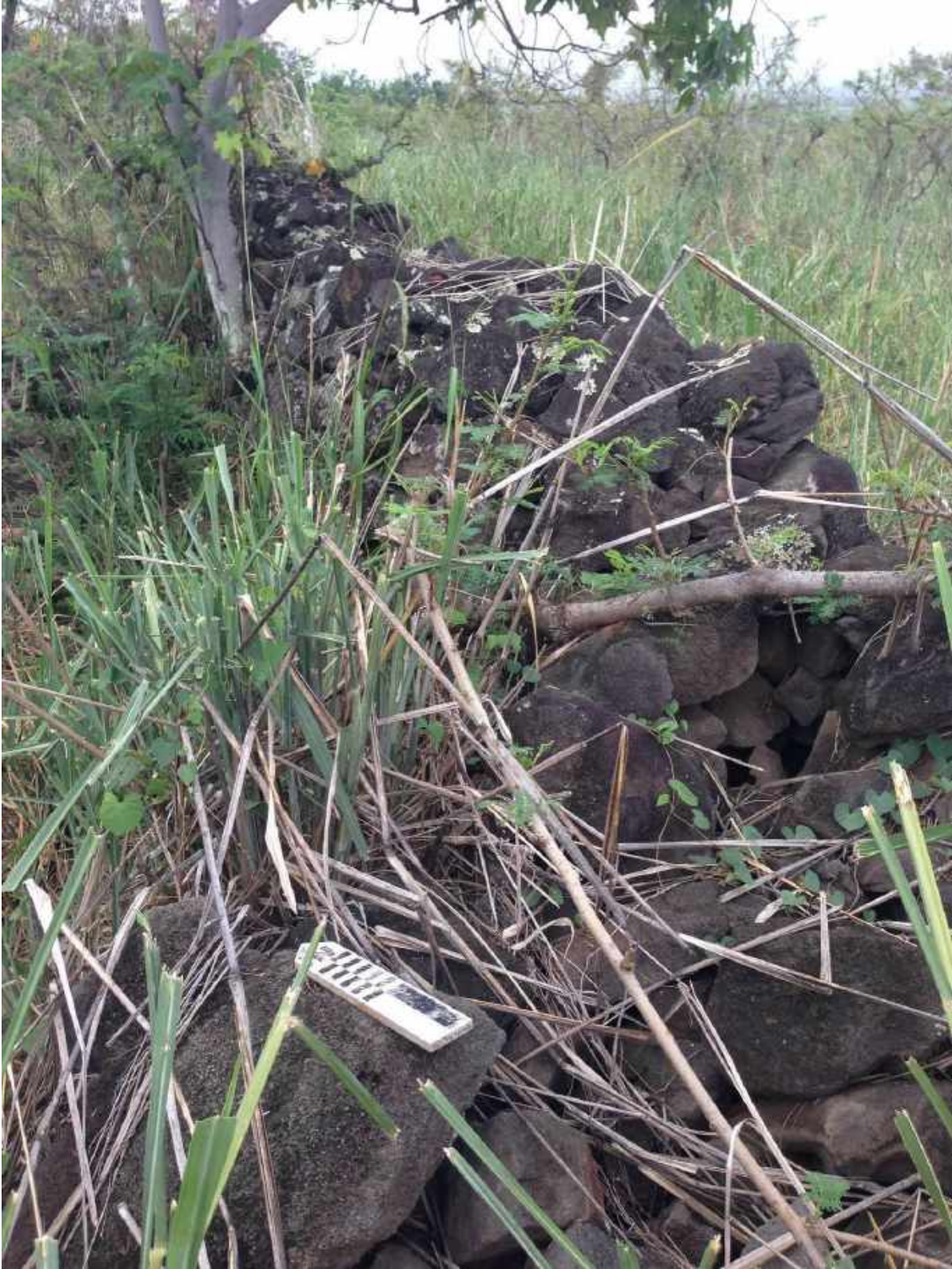
Figure 69: Photograph of Site 31182 Feature 2 South End Showing Top of Wall Construction, Looking Northeast.
