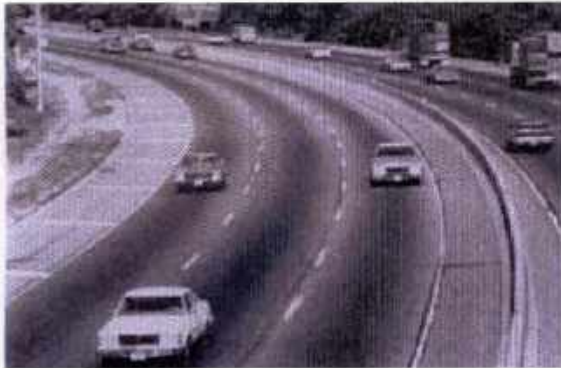
Level of Service A: Free-flow traffic with individual users virtually unaffected by the presence of others in the traffic stream.
