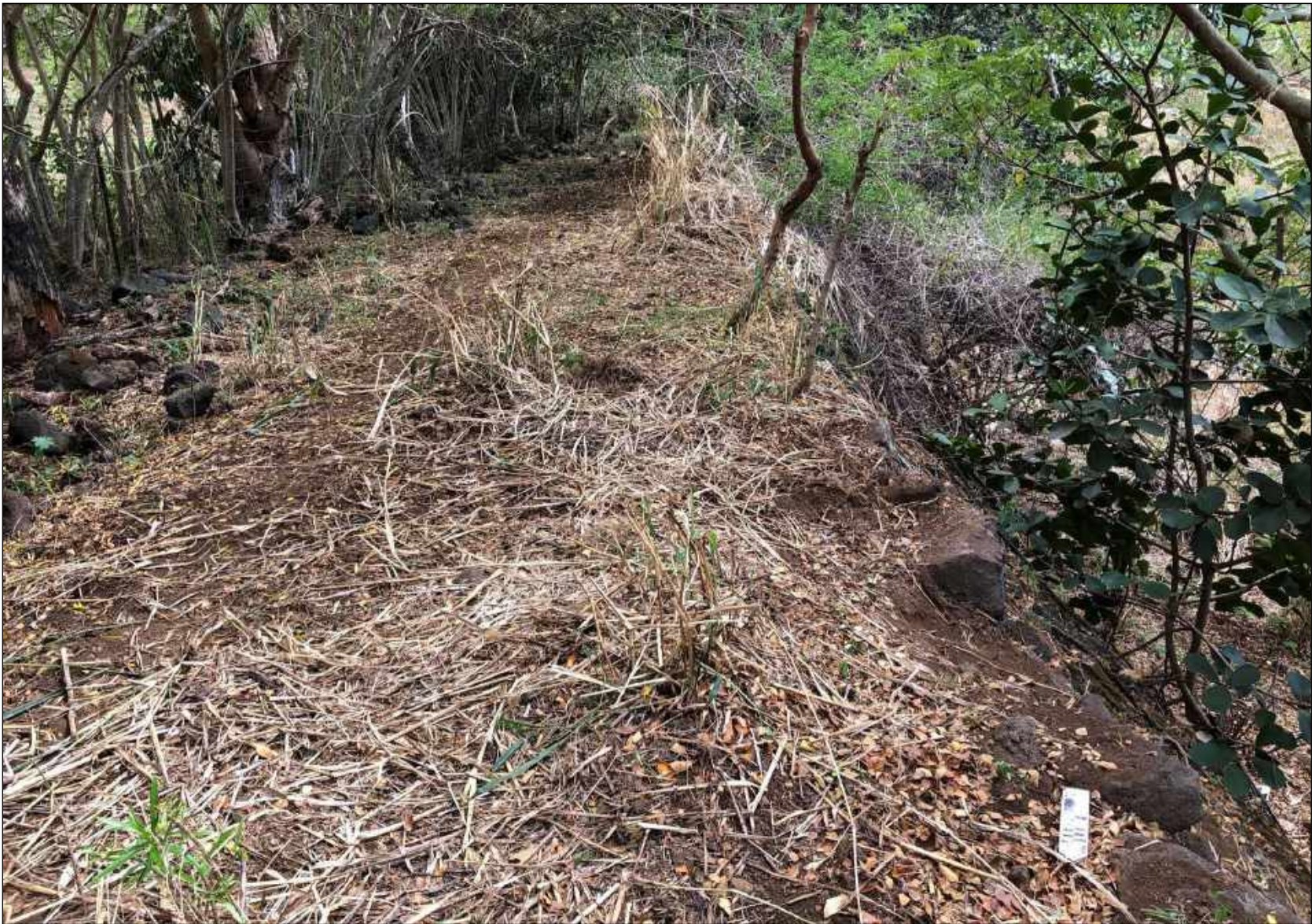
Figure 58: Photograph of Site 30592 Railroad Berm Rail Bed, Looking South.
