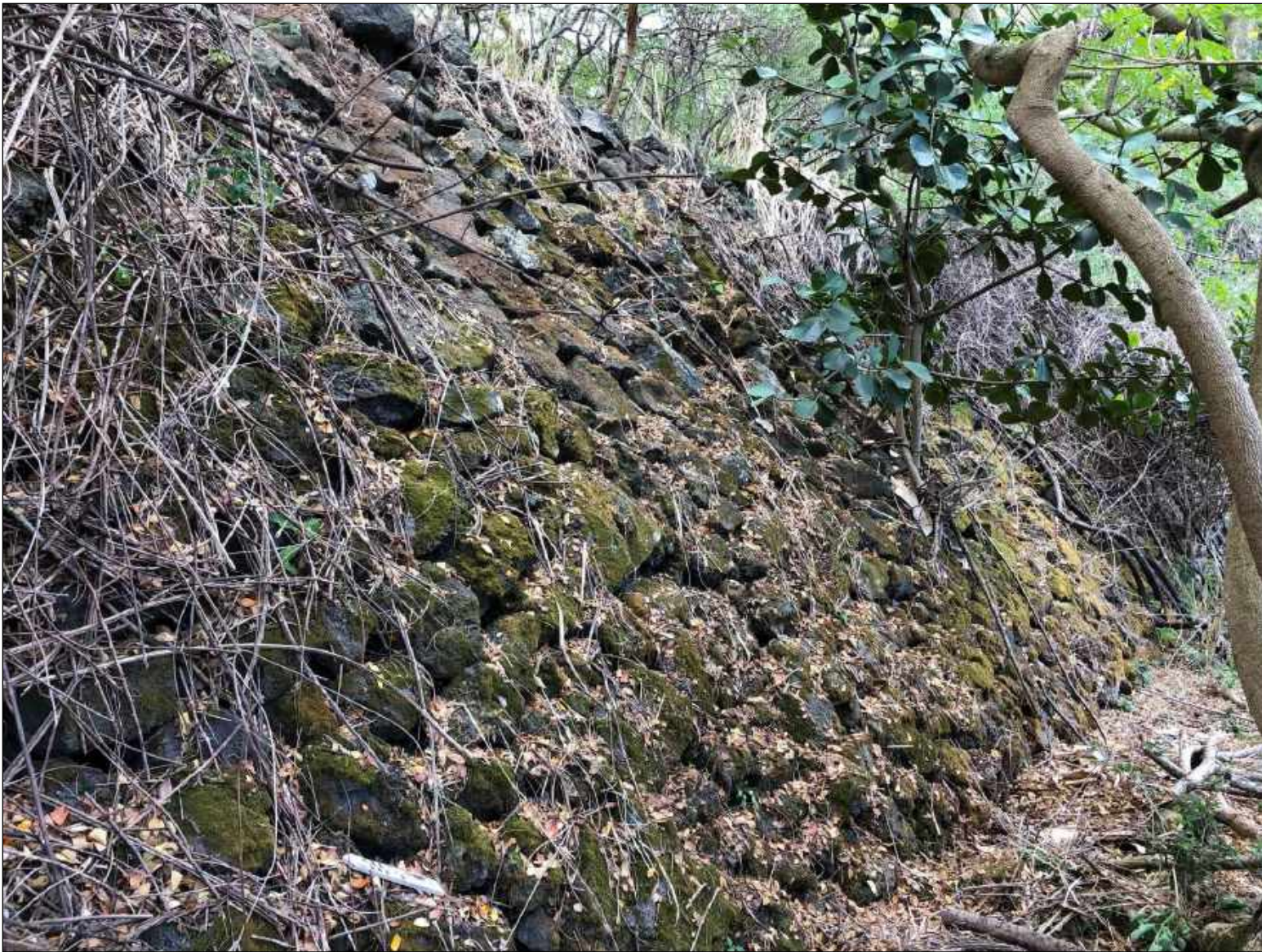
Figure 59: Photograph of Site 30592 Railroad Berm Retaining Wall, Looking Southeast.
