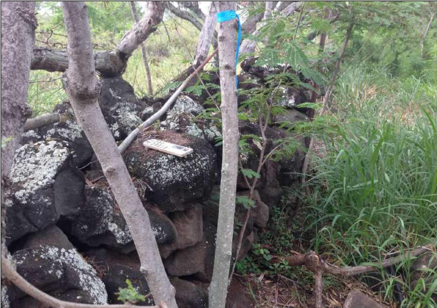
Figure 67: Photograph of Site 31182 Feature 4 South End Showing Wall Construction, Looking North.
