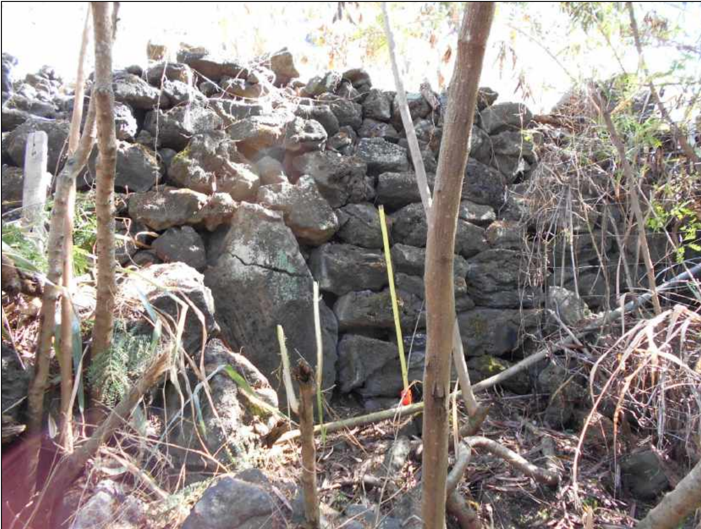
Figure 18: Photograph of Site 30592 Looking East.
